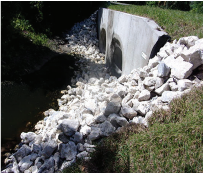
Neighborhood Drainage Improvements
