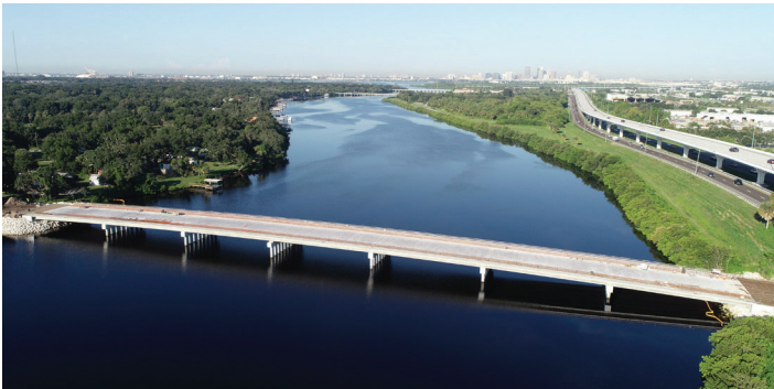
The Maydell Drive bridge connects the Progress Village community to Adamo Drive, and provides connections east and west to Tampa and Brandon.
