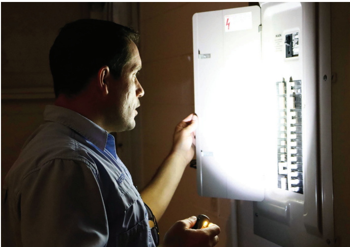
A Development Services inspector conducts an electrical inspection.
