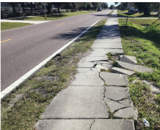
County staff designed and replaced the sidewalk adjacent to the ditch line with reinforcing mat to prevent future erosion issues.
