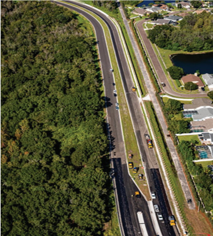
Citrus Park Drive Corridor Improvements
