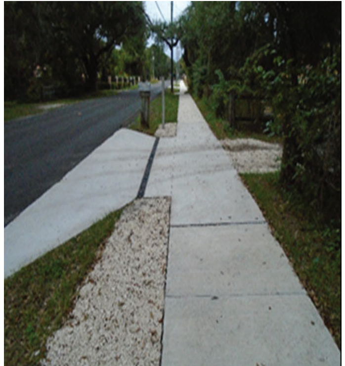
Sidewalk Repair Program
