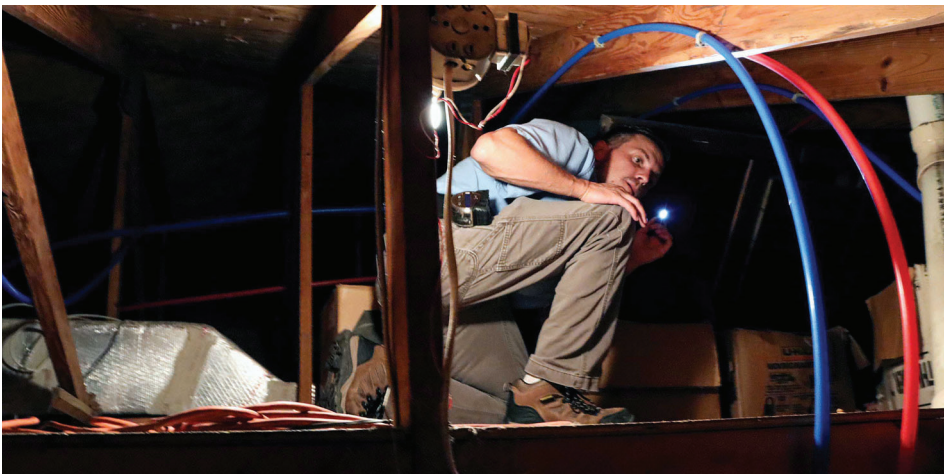
An inspector completes a plumbing inspection.
