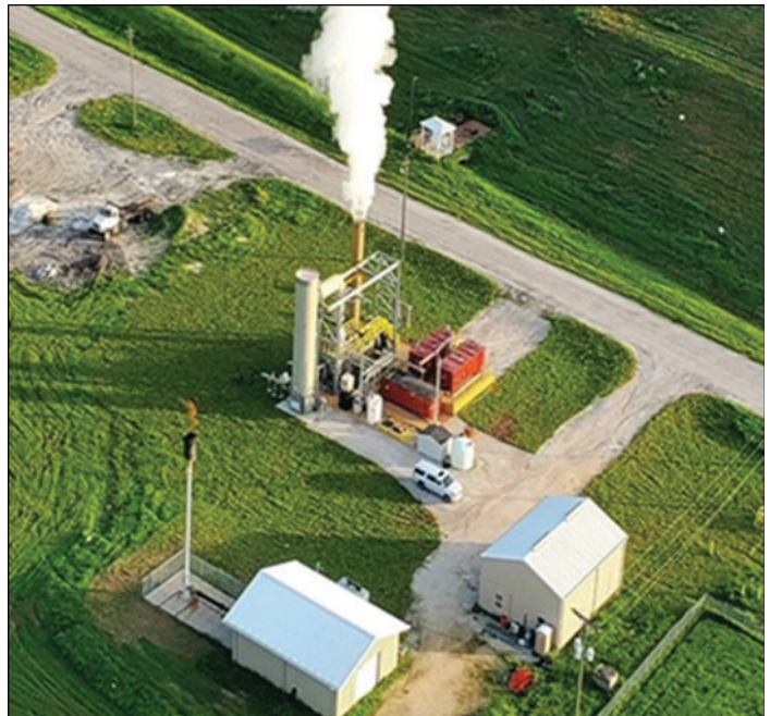
Southeast County Landfill Facility Improvements
