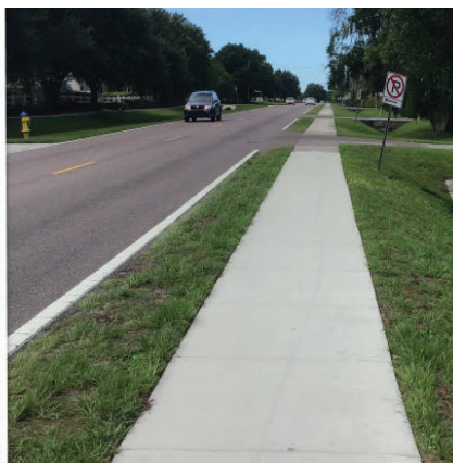
County staff designed and replaced the sidewalk adjacent to the ditch line with reinforcing mat to prevent future erosion issues.
