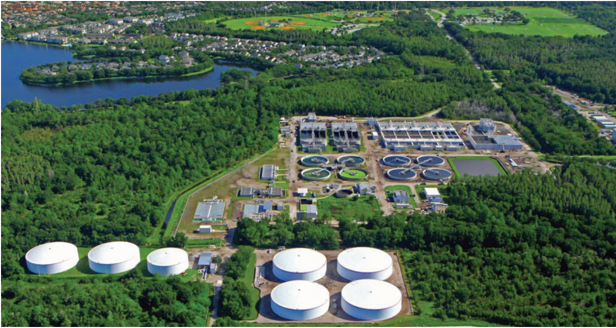
The Northwest Reclaimed Water Facility is shown.
