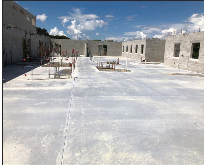
Apollo Beach Fire Station #29 Under Construction
